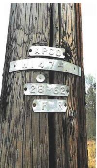
Figures 13 and 14 Structure 28-62: Significant Vertical Pole Cracking
